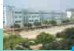
Zhong Shan Plant 2 (China)
